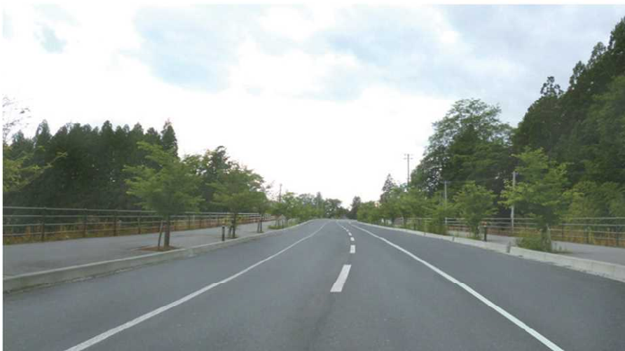
Evacuation road (Symbol Road Image Photo)
